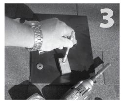
Slide conduit mount into desired position. Remove any nails that conflict with getting the mount flush with front edge of shingle course. Mark cernter for drilling.
