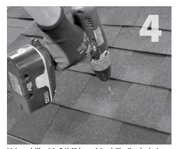
Using drill with 3/16" long bit, drill pilot hole into roof and rafter, taking care to drill square to the roof.
