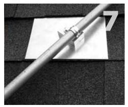
Insert lag through hole in block, and position clamp over conduit. Using drill with 7/16" socket, drive lag until block is tight.
