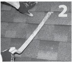
Lift composition roof tile with roofing bar, just above placement of conduit mount.
