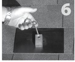
Lift shingle and slide conduit mount into place. Prepare lag bolt with sealing washer and single hole clamp (not included) as shown. Insert lag through hole in block, and position clamp over conduit.
